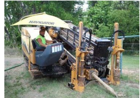
A member of a Peoples Telephone Cooperative construction crew installs fiber in Canton, Texas.
